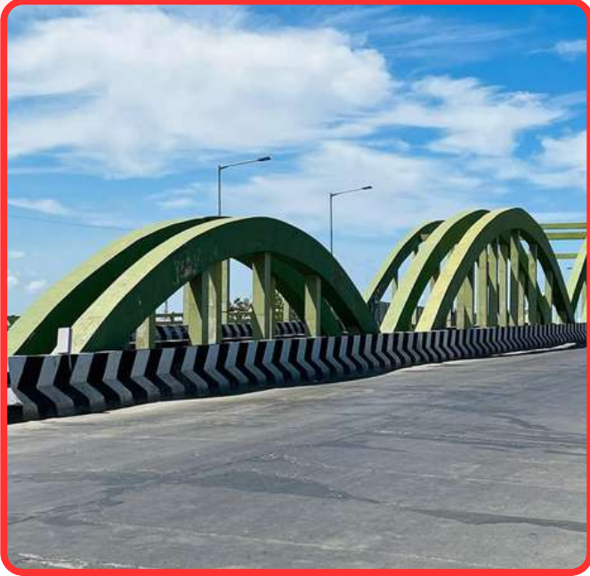
DECK SLAB BRIDGE
